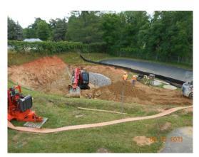
The close of week 14 saw the shoring wall blocks stacked into place and work on leveling the bottom of the site where the process sludge tank will be located. The bar in picture 3 would seem to be the center point of the future tank.
