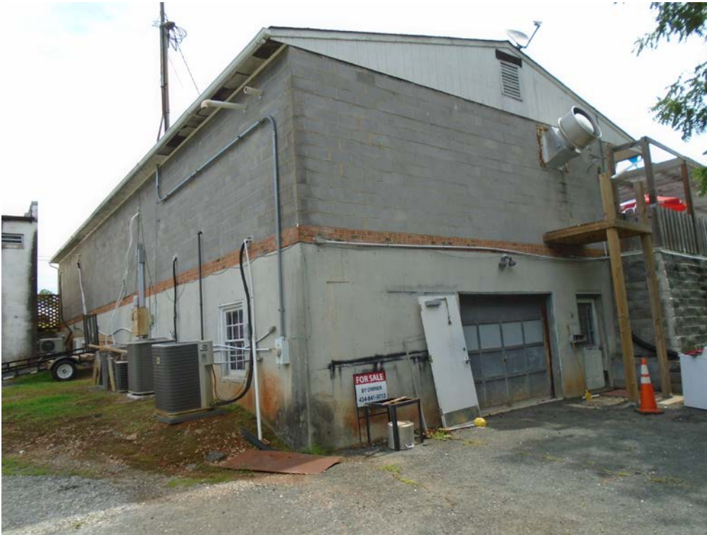
View of the south end of the building
