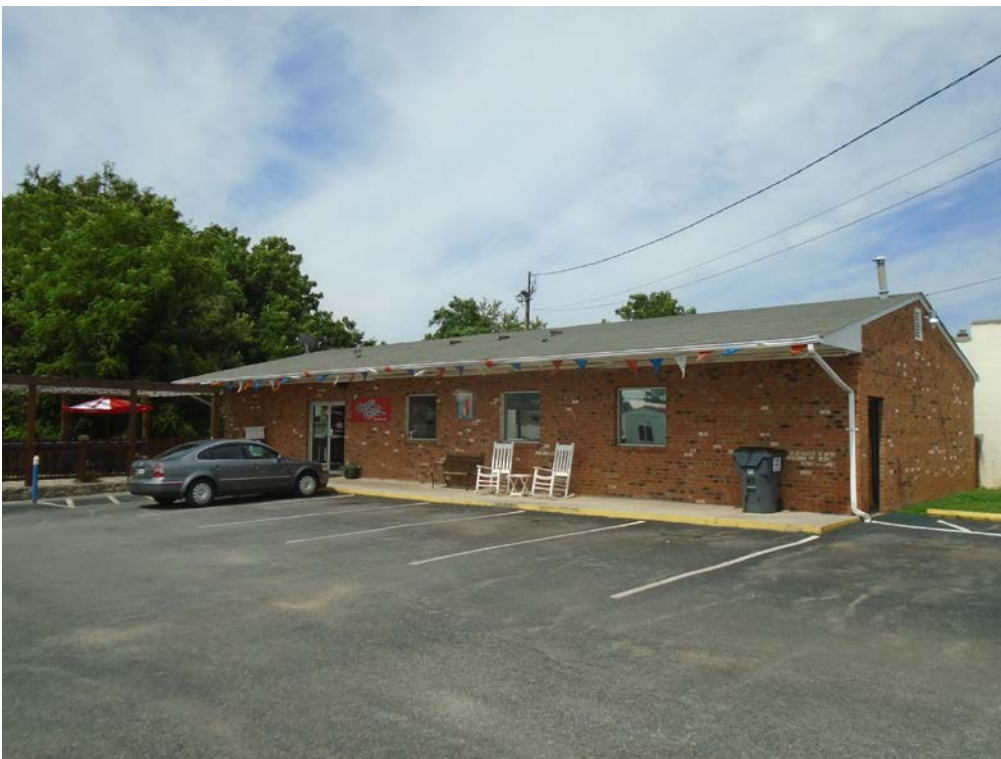
Front view of the building
