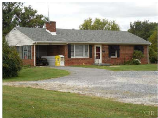
View of office building
