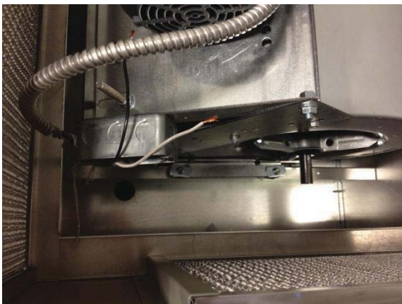
INSTALLED AC POWER WIRING
