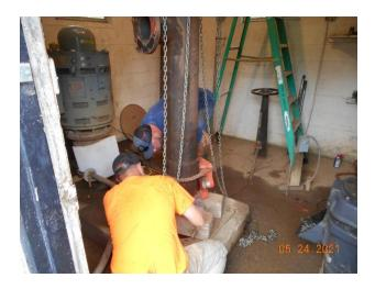
Of most importance in May was the replacement of one of the River Raw Water Pumping Stations pumps due to failure. The drive motor that failed was decades old. It, however, was not clear if the motor itself caused the loss or if the pump has caused the issue. The motor failed, and while in the construction process, the raw water pumping station is not to see upgrade activity until after the first of 2022.
