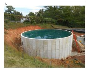
The final leak test on the Sludge Tank was done by completely filling (Pic A) the tank and observing in change in the water volume for 48 hours. No noticeable change was notice so backfilling around the tank was begun. First the blocks acting a the retaining wall were removed (Pic B) and backfill added and compacted (Pic C). Note that this is
