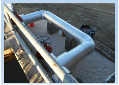
New pipe insulation was put on the raw river water lines coming into the plant, which received the medium and small remaining filter stones.
