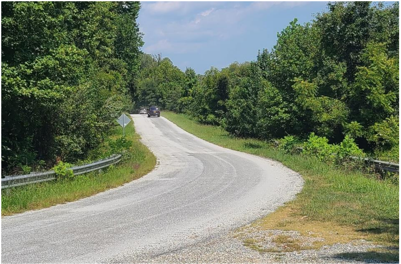
Figure 2- 20' Wide Roadway Ahead of Crest W/Limited Visibility
