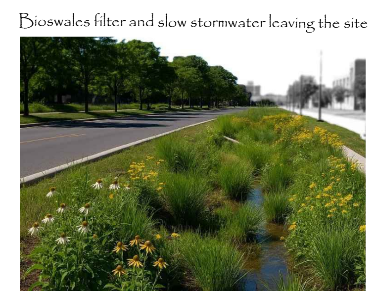
Bioswales filter and slow stormwater leaving the site
