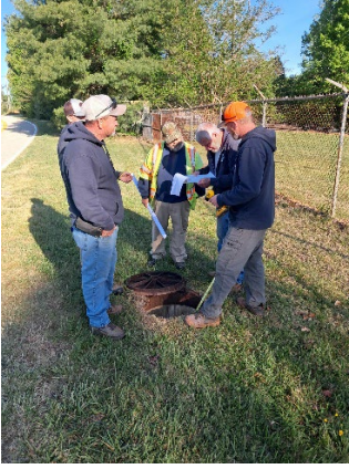
Pulling the pump at 60 west pumping station
