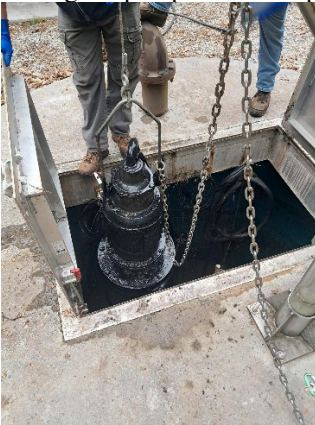
Replacing the gearbox seal at wastewater facility
