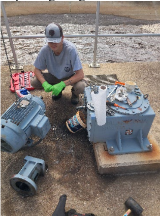
Replacing the gearbox seal at wastewater facility
