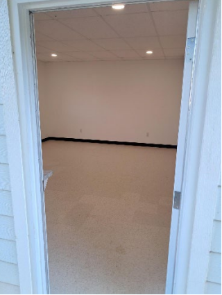
Floor in new building at Maintenance shop.
